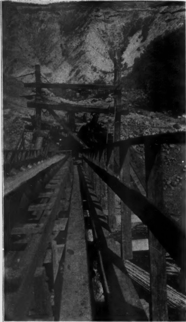
View of Inclined Conveyor. Cedar Grove
